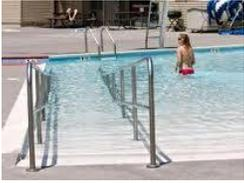
**Sloped Entries** – Sloped entries are similar to ramps that are used on dry land. They are expensive to install but virtually maintenance-free once they are in place.
